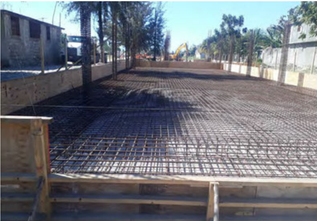
Finished reinforcement awaiting the pouring of concrete
