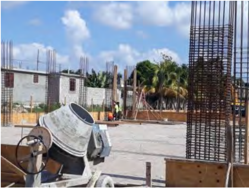
Les Cayes Works – Feb/2020
