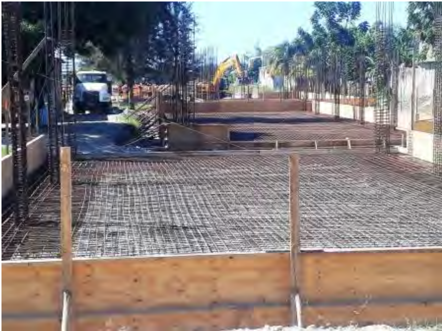
Finished reinforcement awaiting the pouring of concrete
