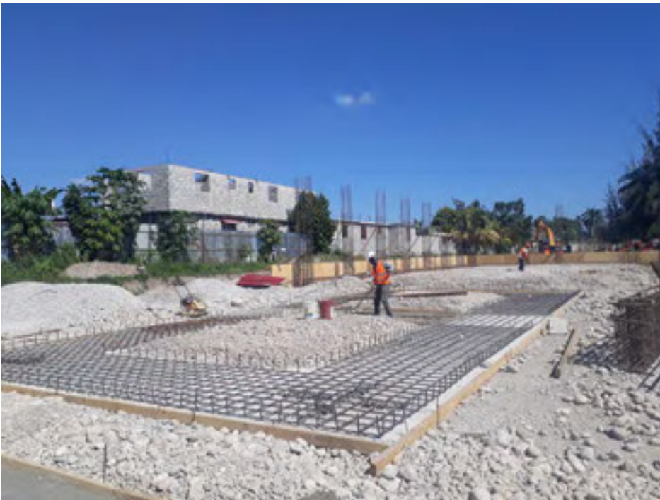
Finished reinforcement awaiting the pouring of concrete
