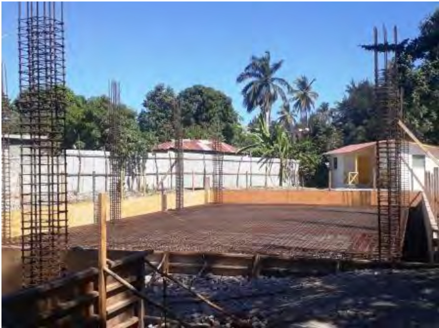
Finished reinforcement awaiting the pouring of concrete
