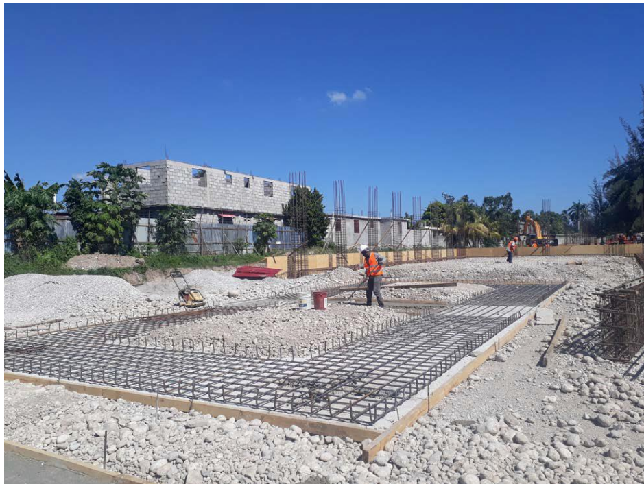
Finished reinforcement awaiting the pouring of concrete
