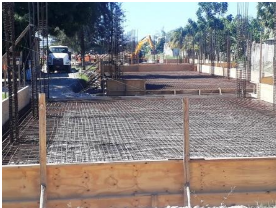
Finished reinforcement awaiting the pouring of concrete
