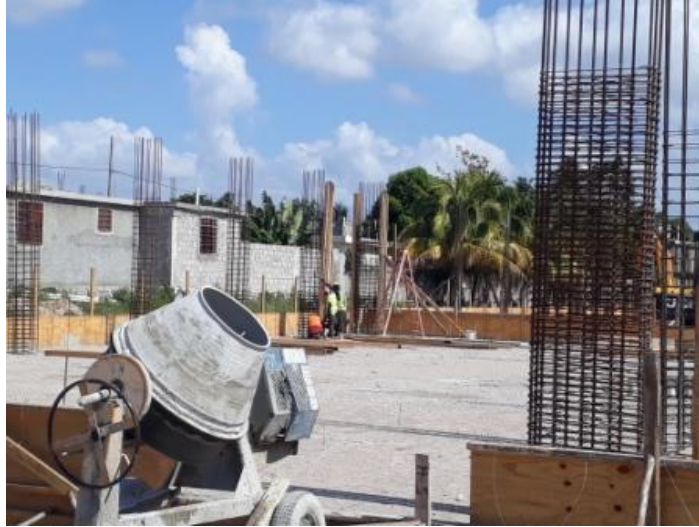
Les Cayes Works – Feb/2020
