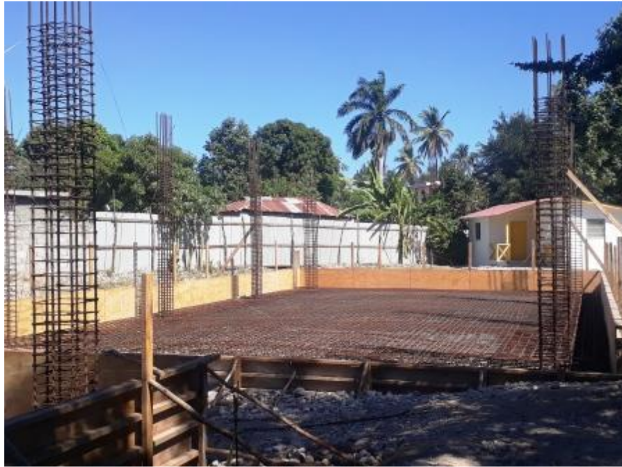
Putting in place concrete of cleanliness and starting of the reinforcement
