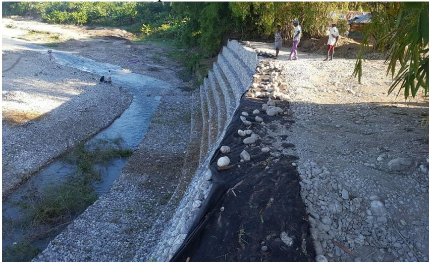
Gabion protective wall in the river
