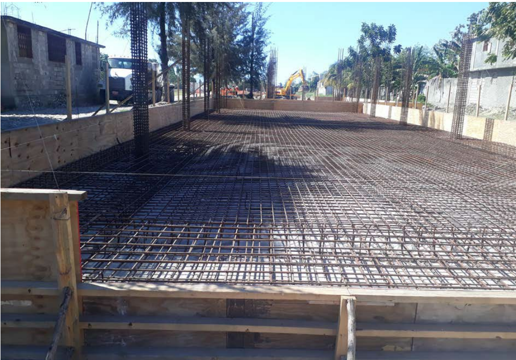
Finished reinforcement awaiting the pouring of concrete
