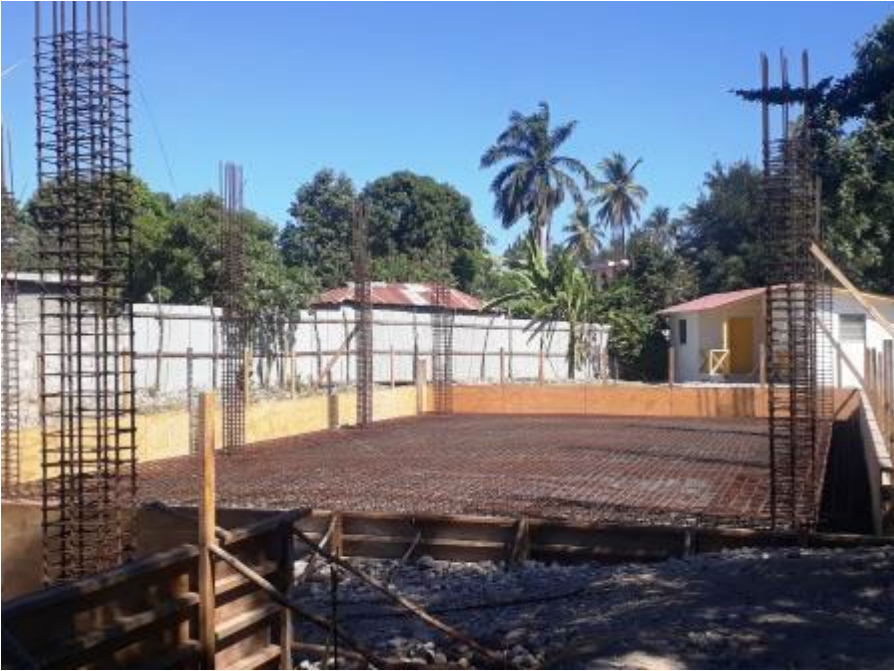
Finished reinforcement awaiting the pouring of concrete
