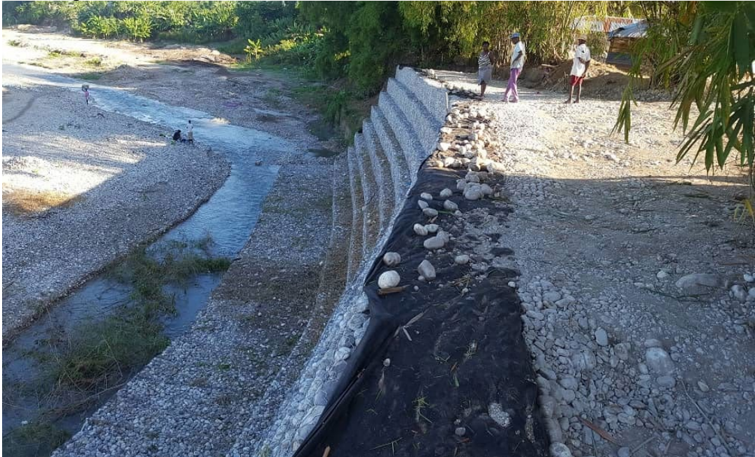
Gabion protective wall in the river
