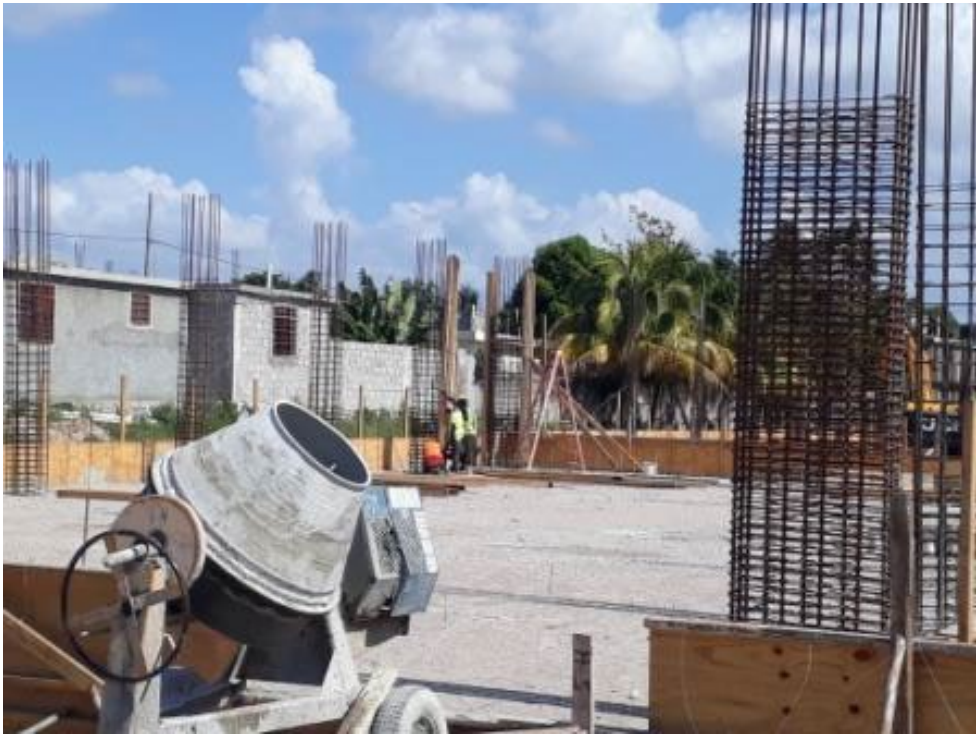
Les Cayes Works – Feb/2020
