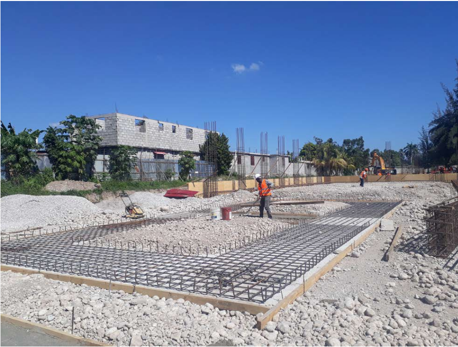
Finished reinforcement awaiting the pouring of concrete
