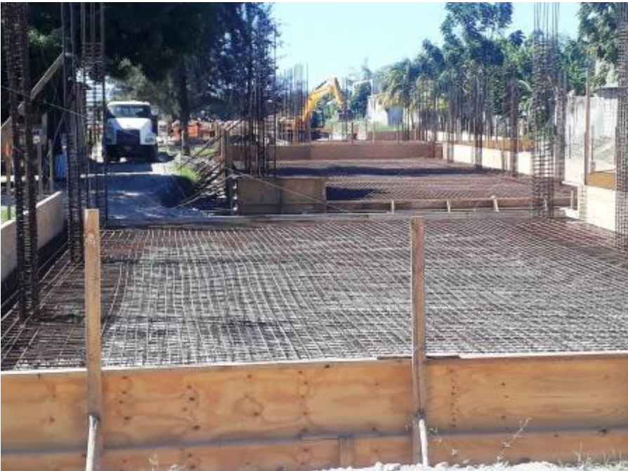
Finished reinforcement awaiting the pouring of concrete
