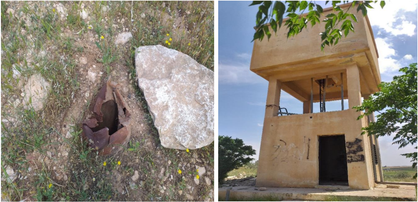
Figure 10: Nassib Alfayiz groundwater well
