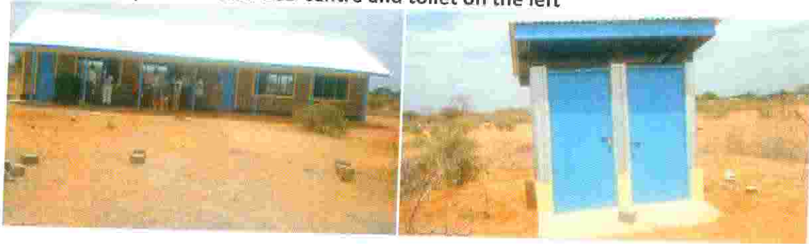
Fig 9: Recently constructed ECD centre and toilet on the left
