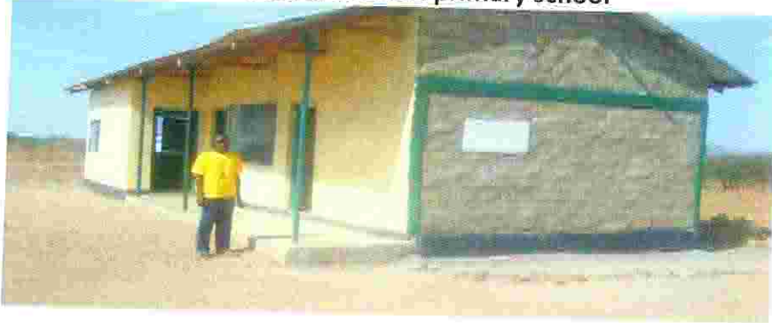
Fig 10: the new office block at Letea primary school
