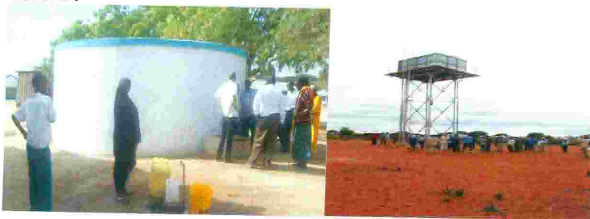
Figs 8: concrete and steel water tanks constructed at Dadaad primary and secondary schools respectively
