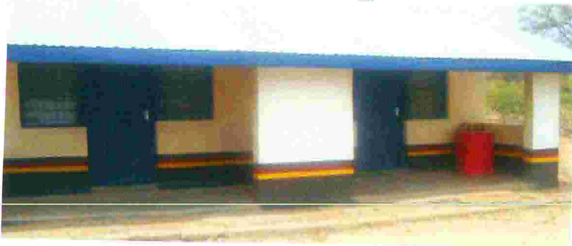
Fig 4: Newly build police Officers' houses in Lokichoggio
