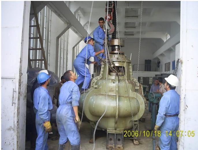
FAO trained MoA engineers installing a water pump
